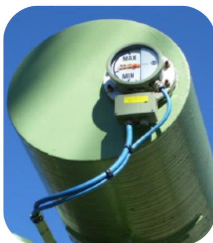
Figure 1 – Oil level sensor on the transformer conservator [4]
